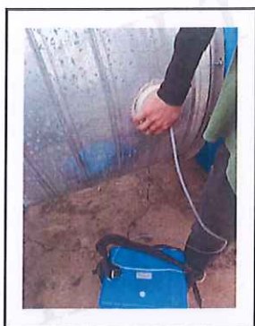
注塑成型、移印、洗网、回流焊、波峰焊、补焊、擦拭废气处理前
